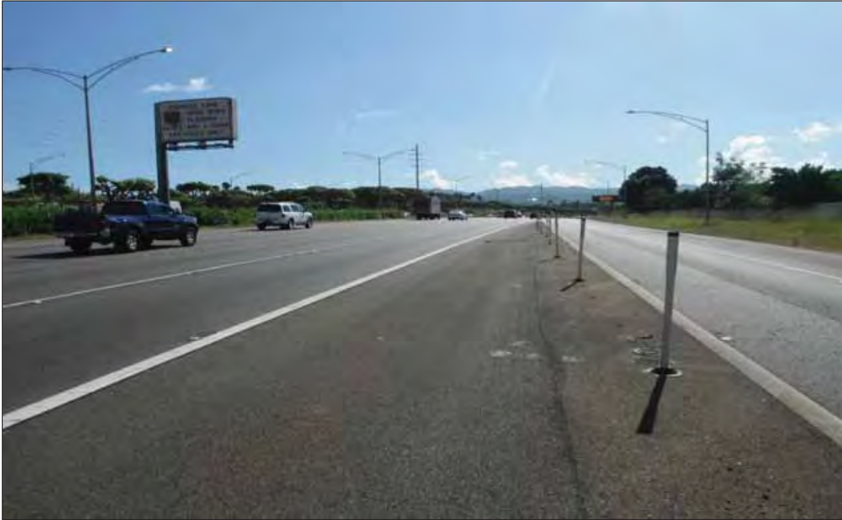
View to Northeast
